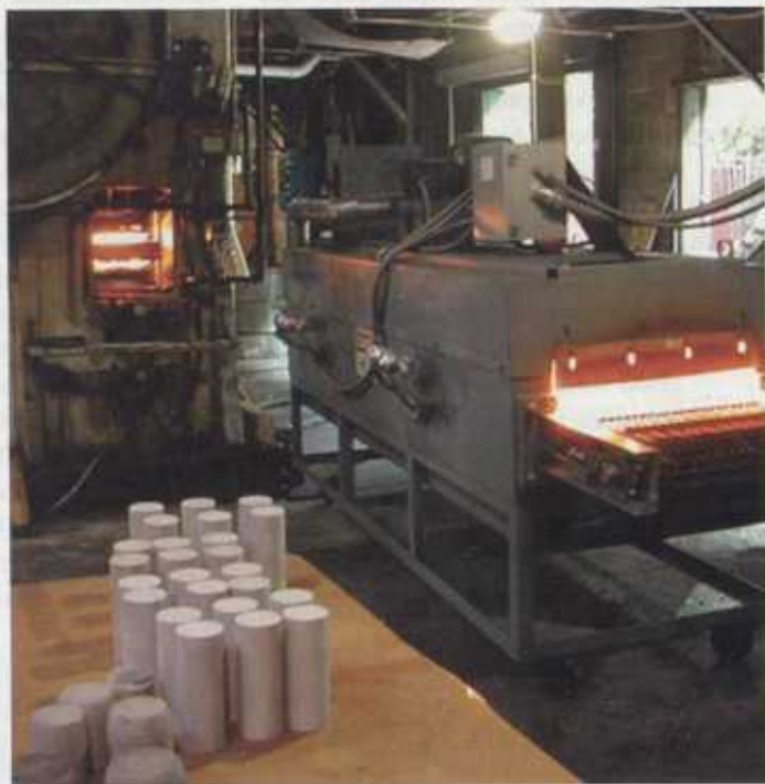
Queen City Forging's Rapid Infrared heating furnace preheating aluminum billets
